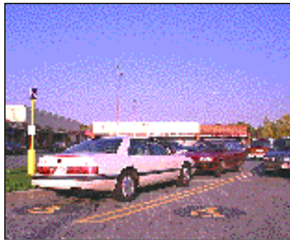
These parking spaces are too narrow and lack a wide access aisle so people who use wheelchairs cannot get out of their vehicle.
